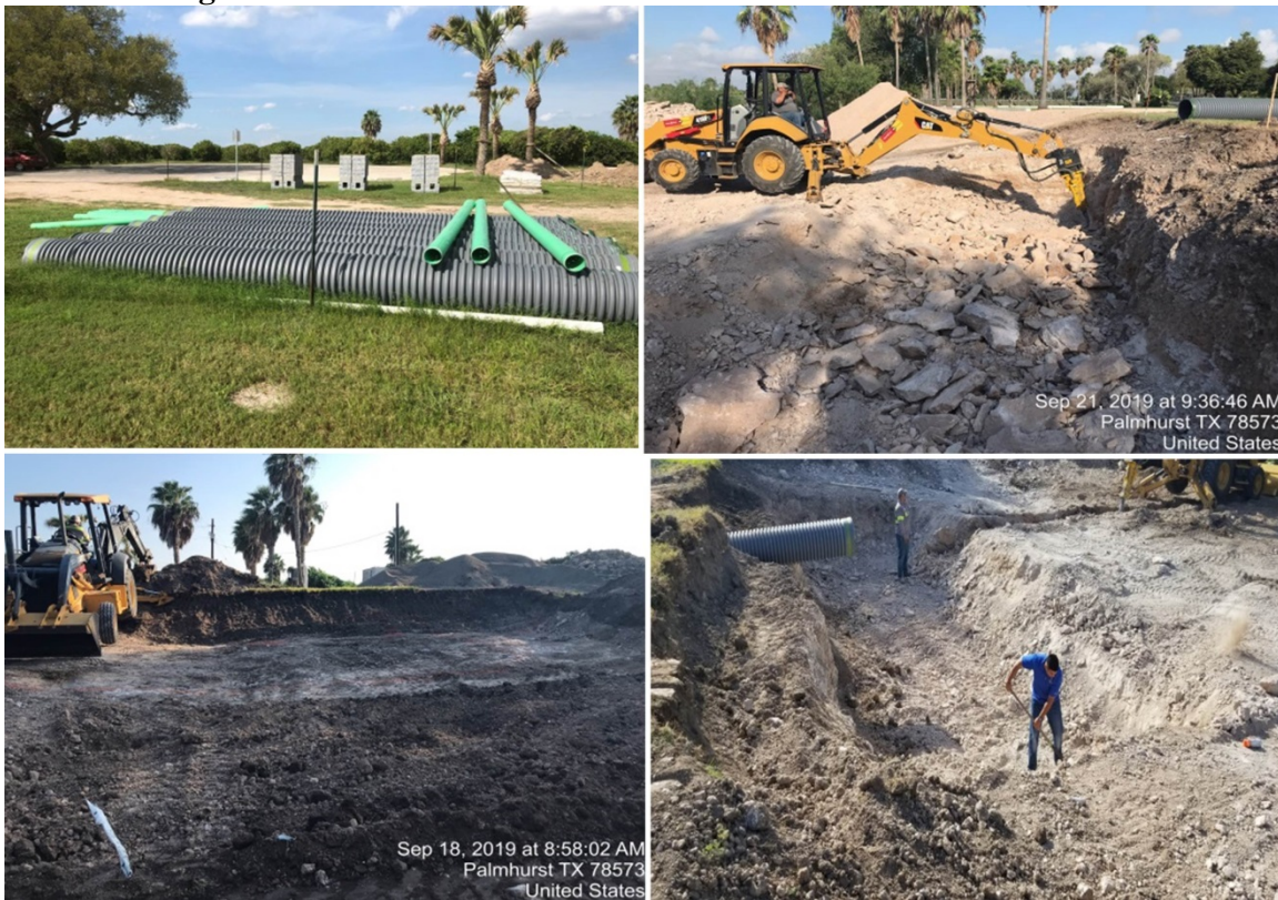
Figure 3. Construction starts at the site and materials used.
