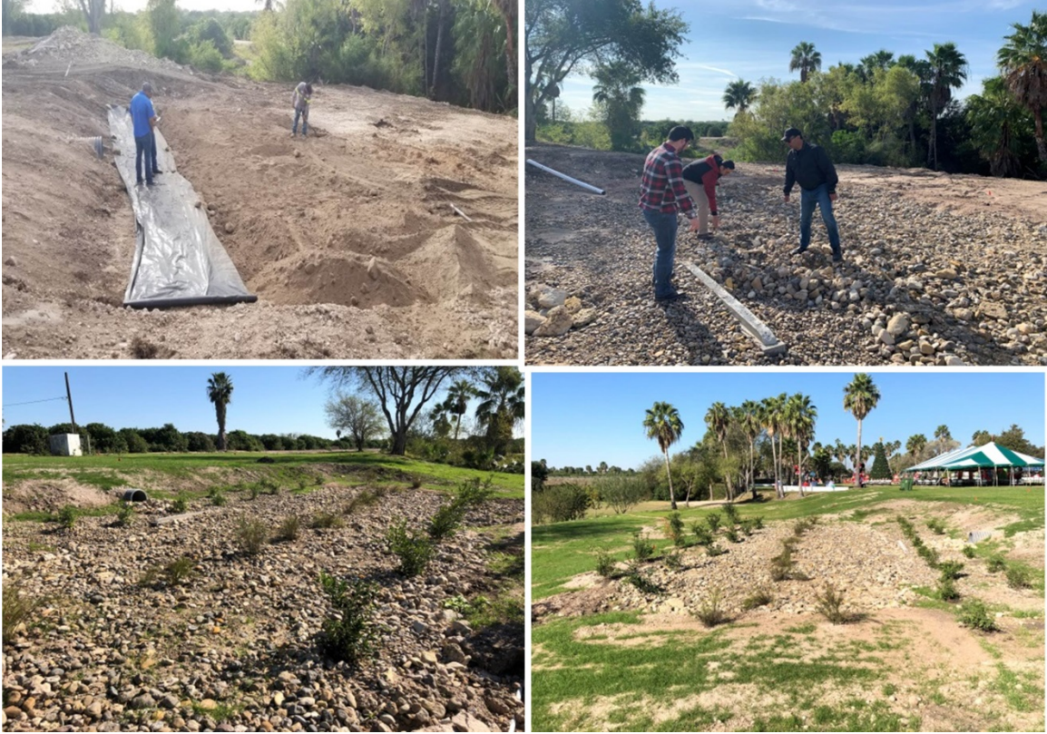
Figure 6. Bioretention cell surface cover and site after construction.
