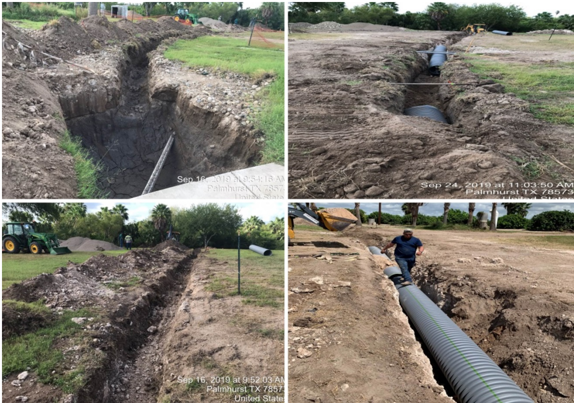
Figure 4. Excavation at the site and pipe installment.
