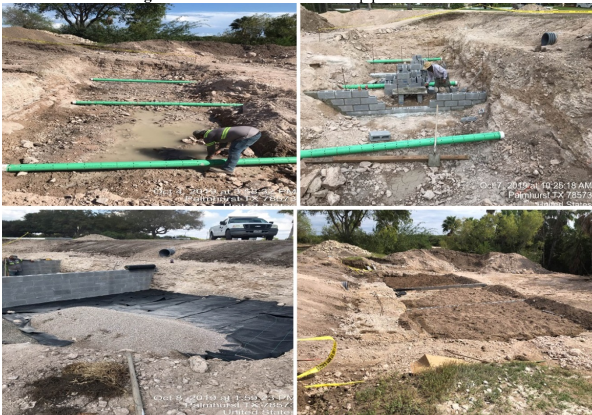
Figure 5. Bioretention three cells build up and different media used for each cell.
