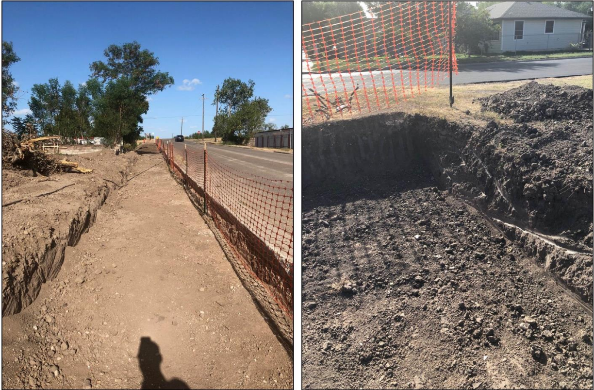
Figure 4. Construction starts at the site.
