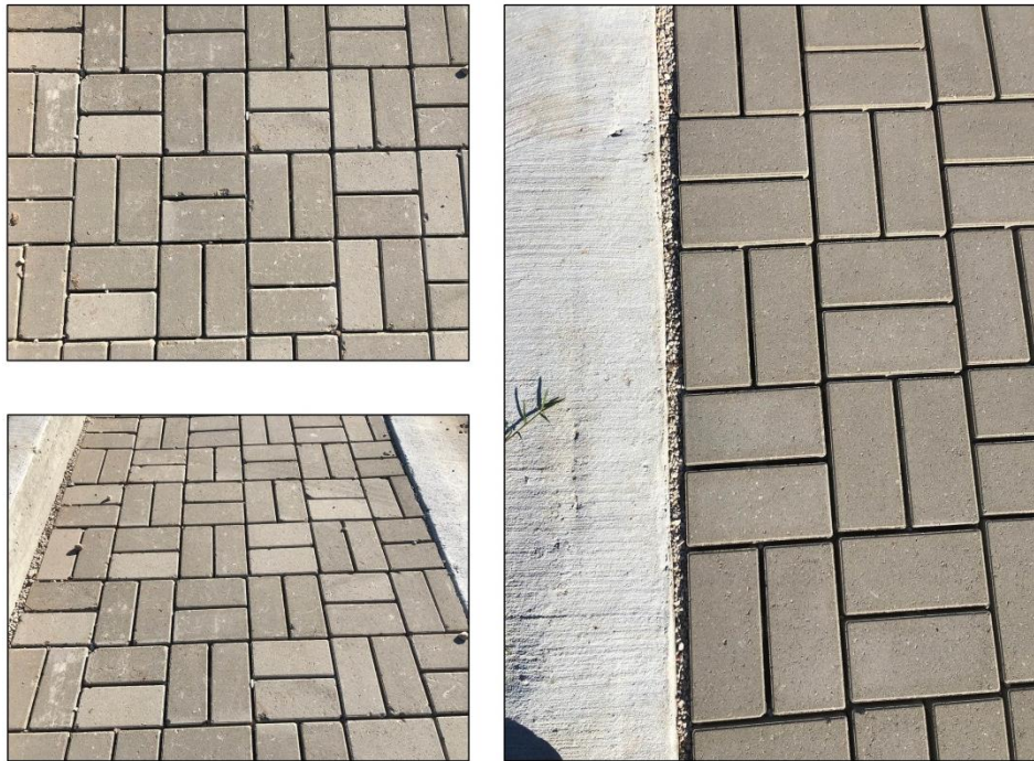
Figure 6. The permeable pavement joints filled with gravel to increase the runoff infiltration.
