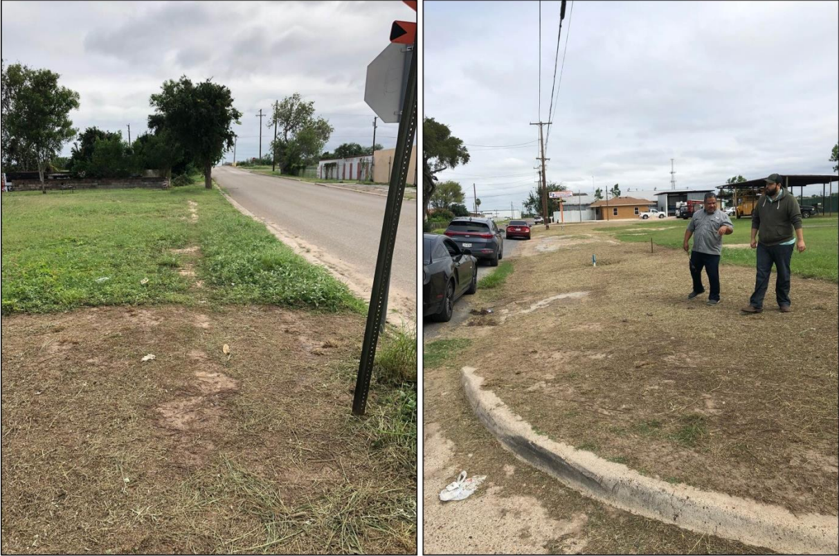
Figure 3. Permeable pavement location and site before the construction starts.
