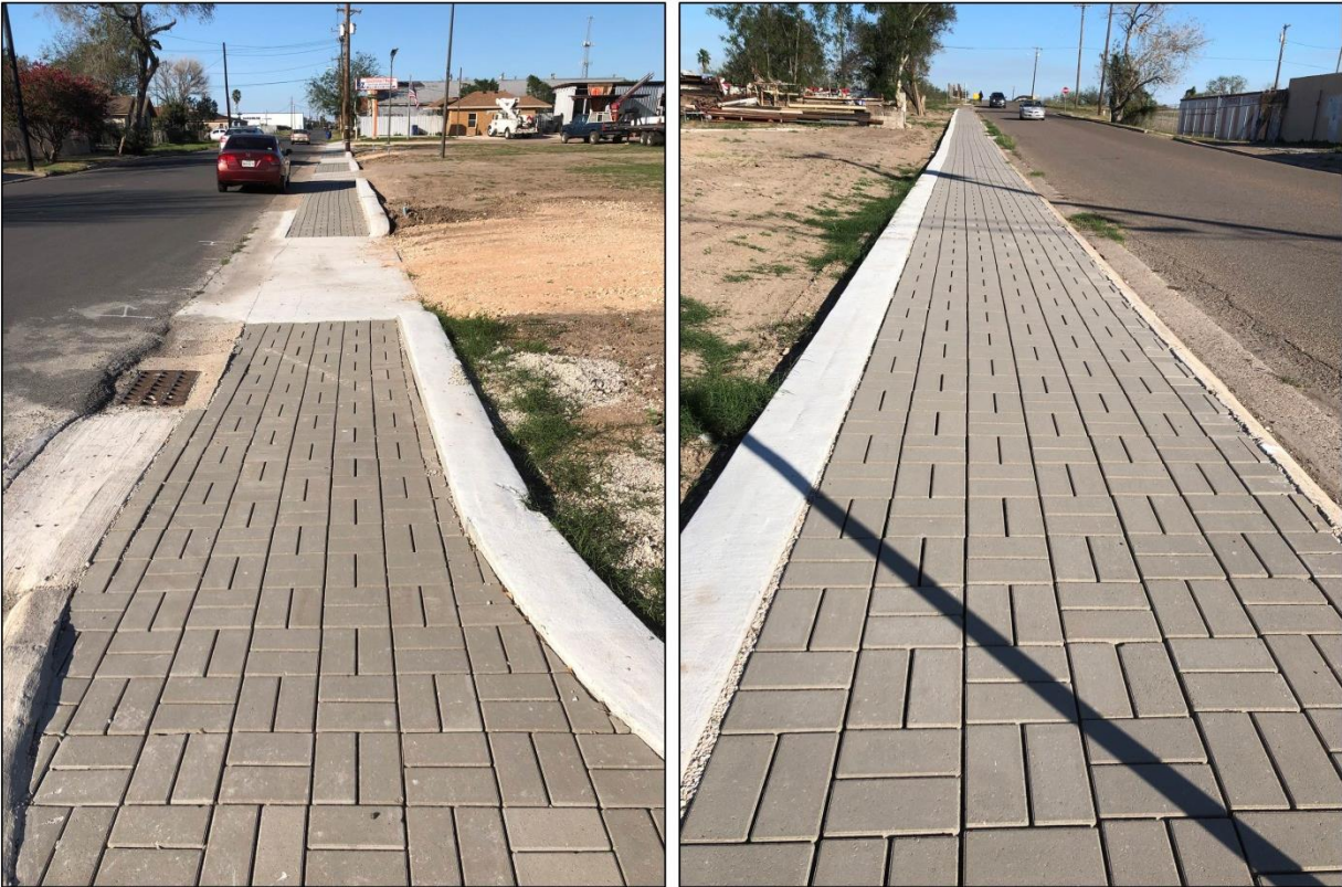
Figure 5. The two sides of the Permeable pavement after the construction.
