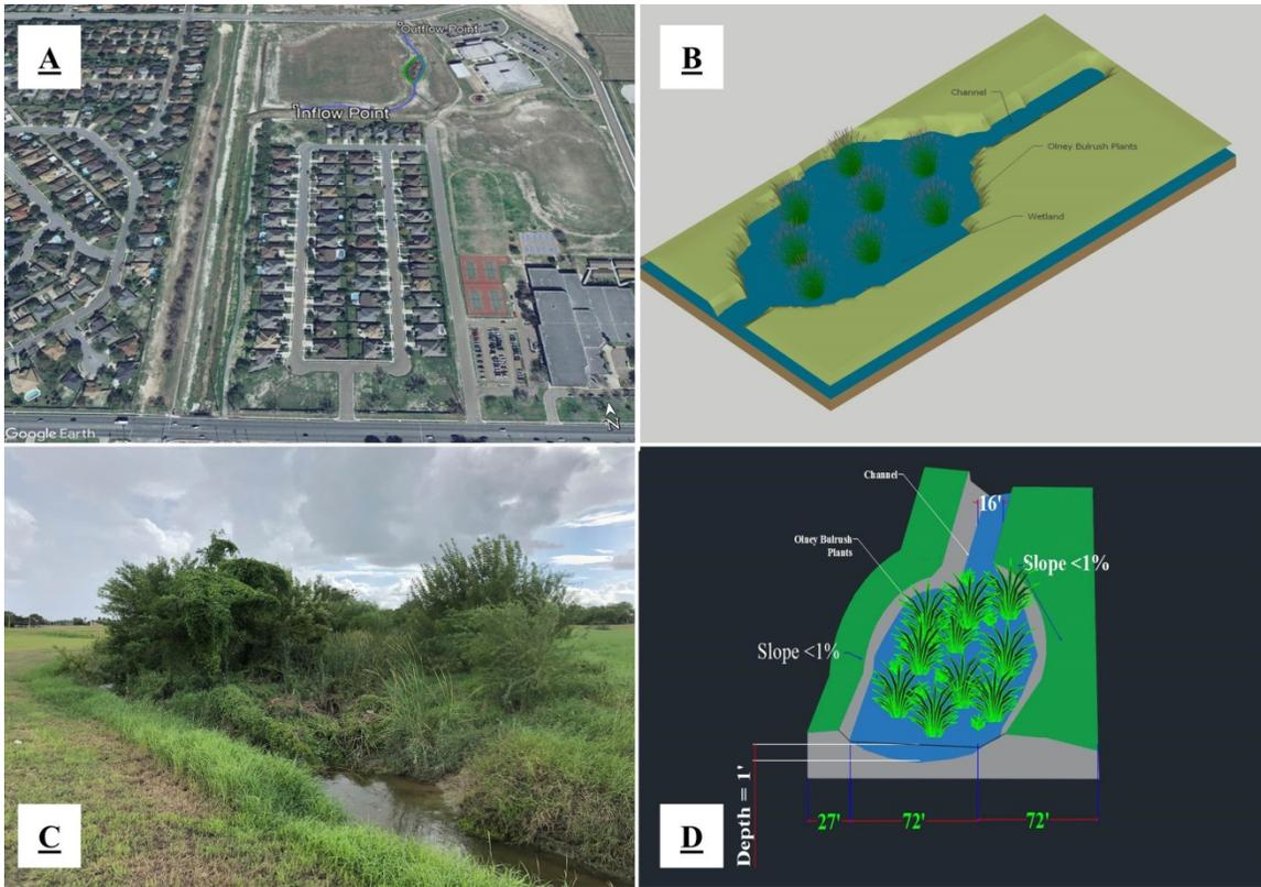
**Figure 3.** Morris Regional Detention Facility (RDF) site: (A) aerial view for the site location, (B) wetland structure, (C) vegetation on the wetland, and (D) cross-section showing the depth and dimensions of Morris wetland.
